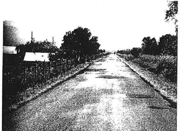
4. Looking west 1.172 Miles from Adams Rd
