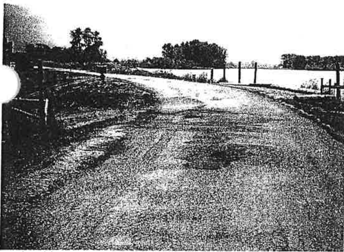
3. Looking west 0.821 Miles from Adams Rd
