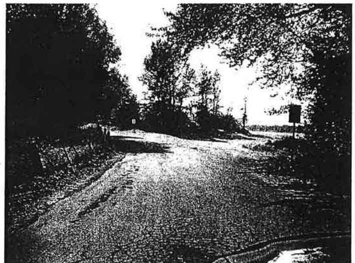
12. Looking west 3.362 Miles from Adams Rd.
